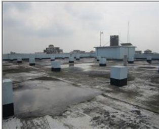
External photo(s) of the production unit(s) Roof top.JPG
