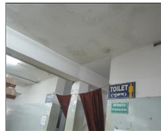
Photo of the sanitary facilities Toilet for male.JPG
